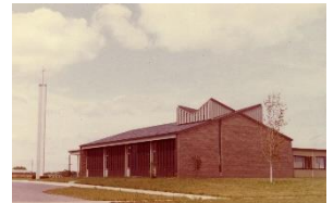
Our original building
